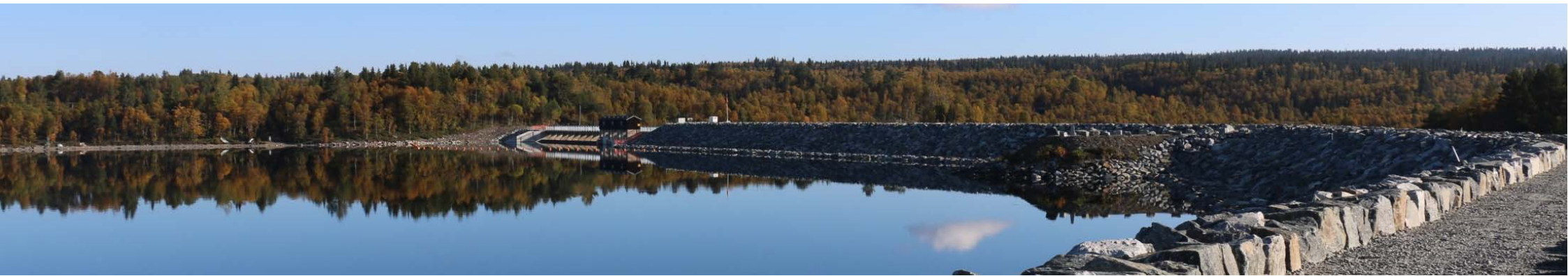
Tisleifjord hydropower plant
